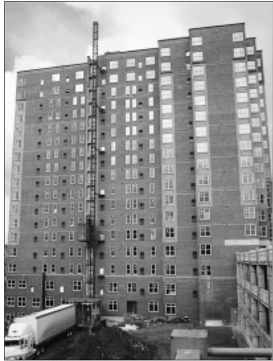
Right: Materials were moved to the interior of the topped-out building via a hoist.
