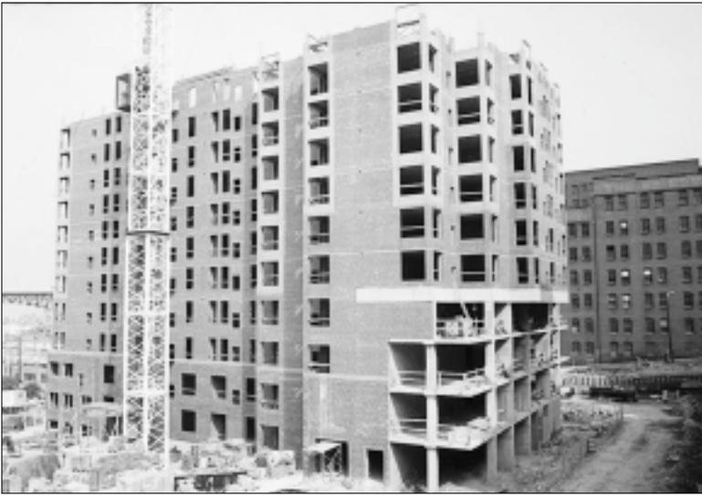
Above: The brick curtain walls were anchored at every floor to the floor planks with special anchors that allow movement vertically but not horizontally. This photo shows work up to the 10th floor, prior to construction of the garage.
